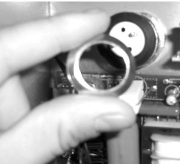
9. Replace retainer nut and finger tighten.
